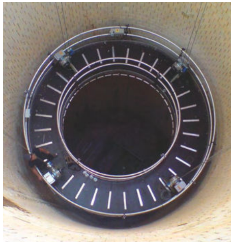
Shaft Access Platform
