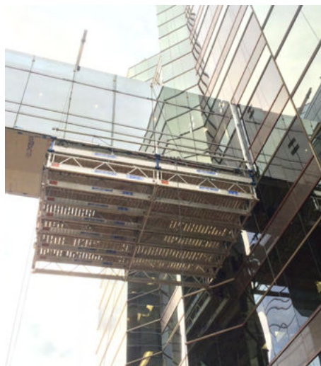
Rolling SSU Deck under Pedestrian Walkway
