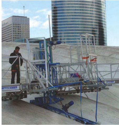
Concrete Shell Roof Access
