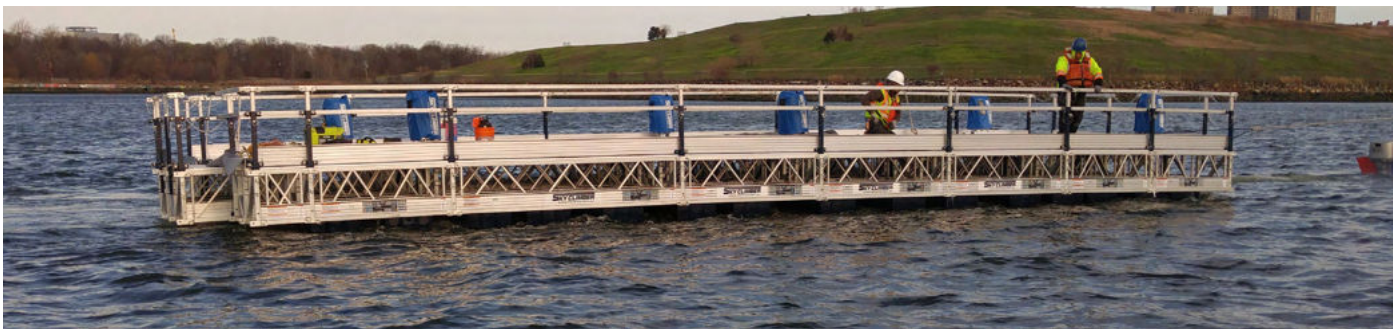
Floating Bridge Maintenance Deck
