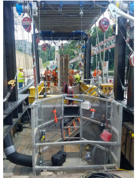
Cofferdam Access Platform
