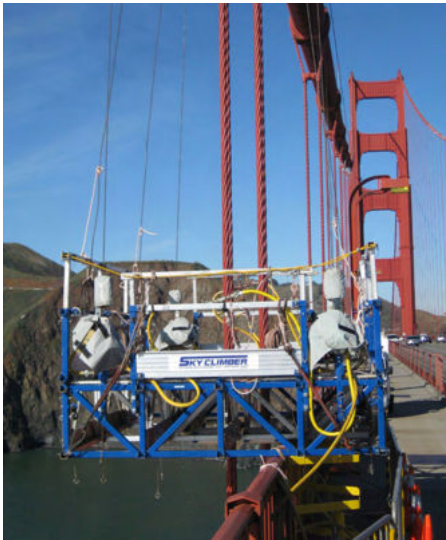
Bridge Cable Maintenance Platform
