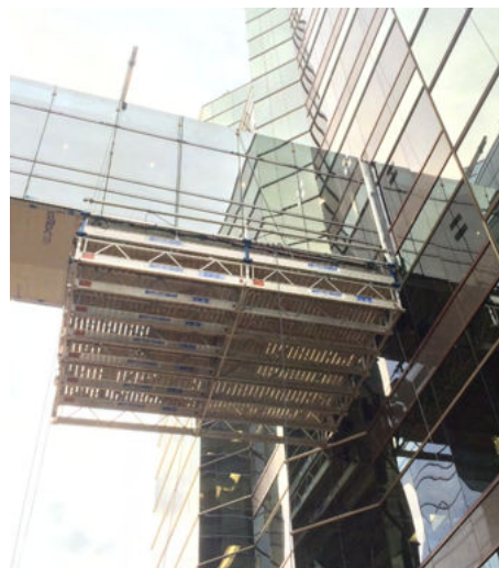
Rolling SSU Deck under Pedestrian Walkway
